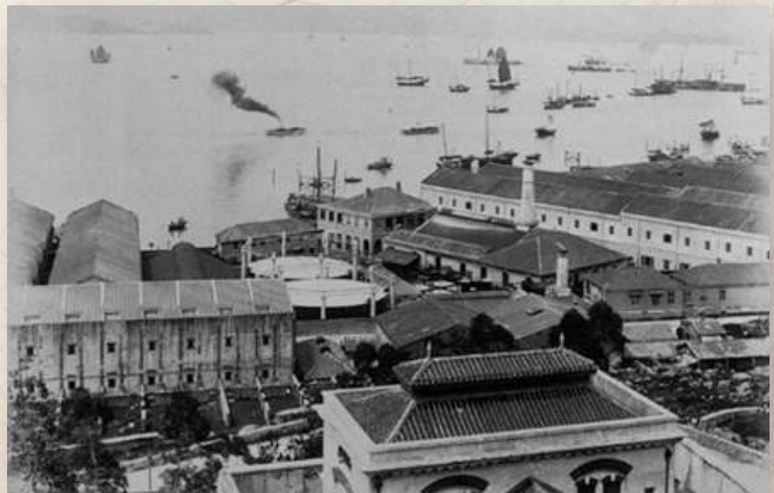
Figure 4: The gasworks in Shek Tong Tsui in the 1880s, the coal sheds are probably the black-roofed building on the left of the gasometers.
