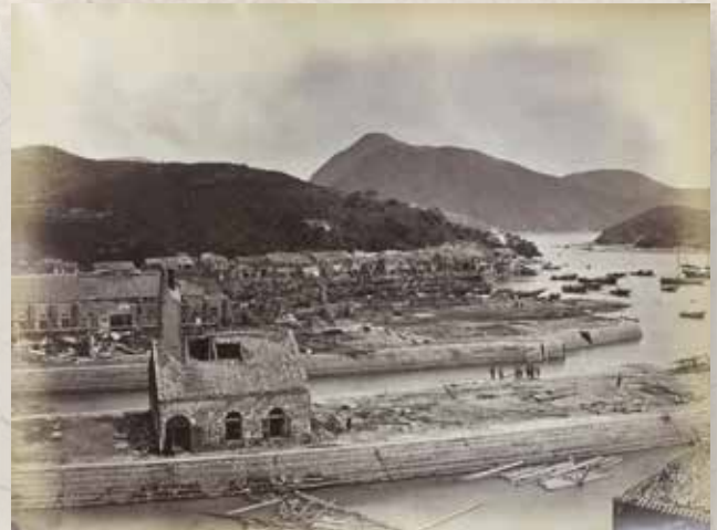
Figure 6: The first boiler and pump house with its typhoon topped chimney
